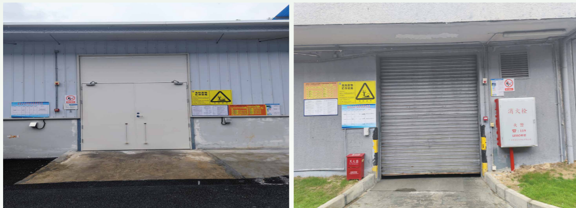
Hazardous waste storage facility
